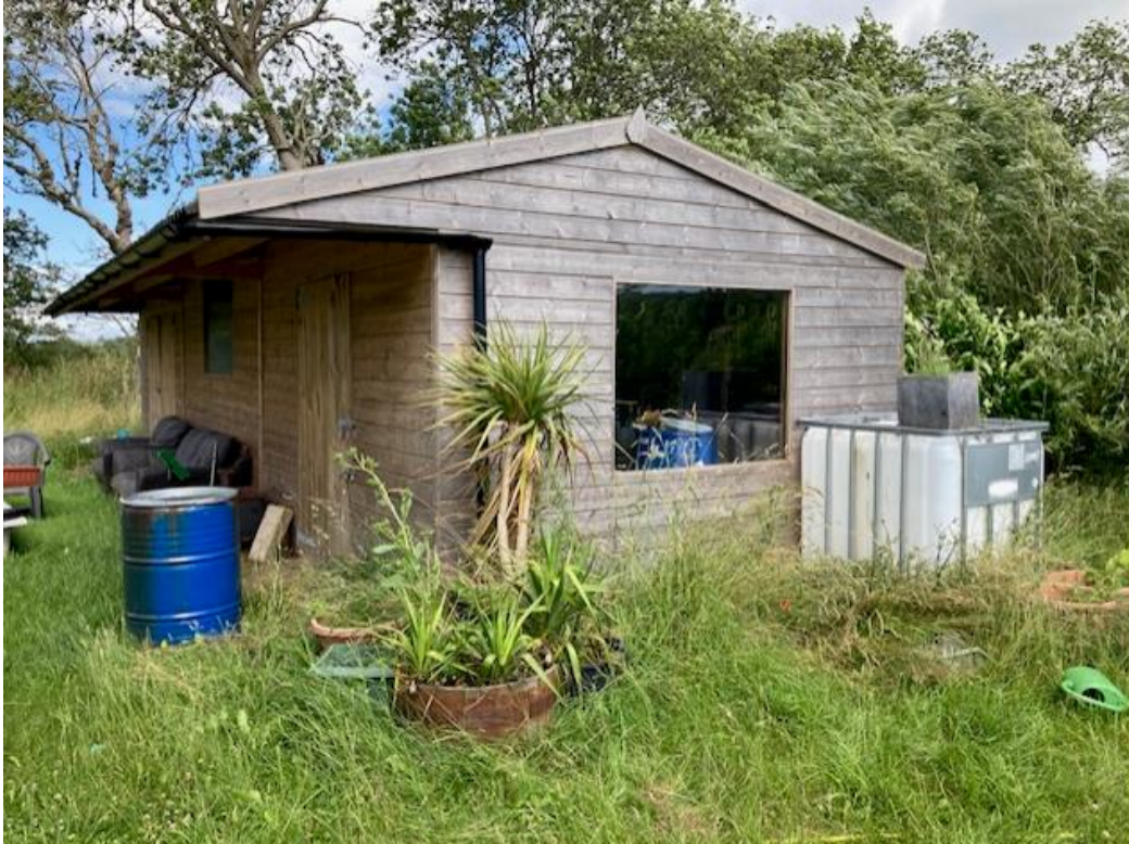
Figure 1: Photograph of shed A.
